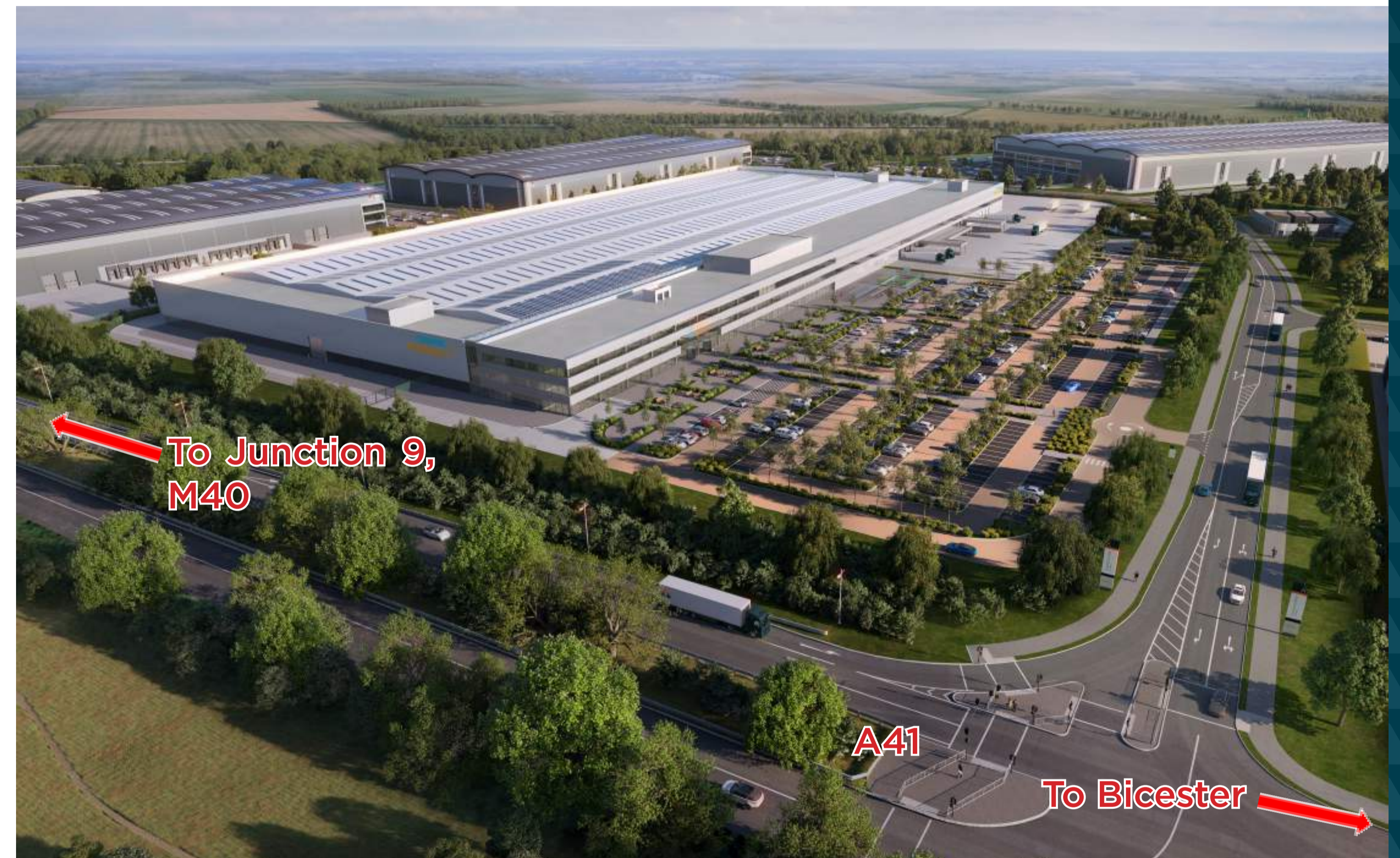
CGI of Siemens Healthineers (under construction)
