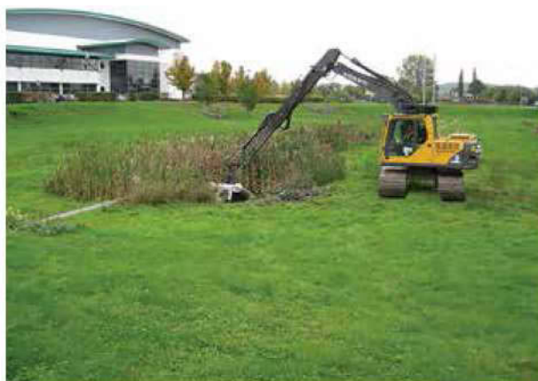
Figure 32.2 De-silting (courtesy Bedford Group of Drainage Boards)
