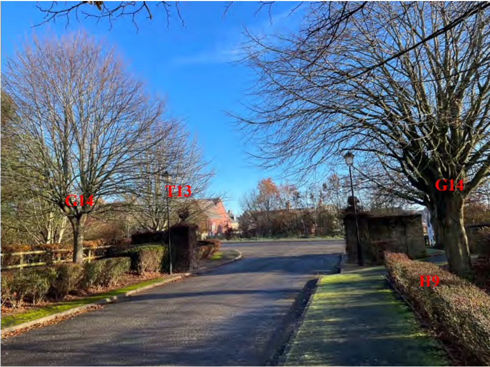
Photoview 8: View looking east at the site entrance.
