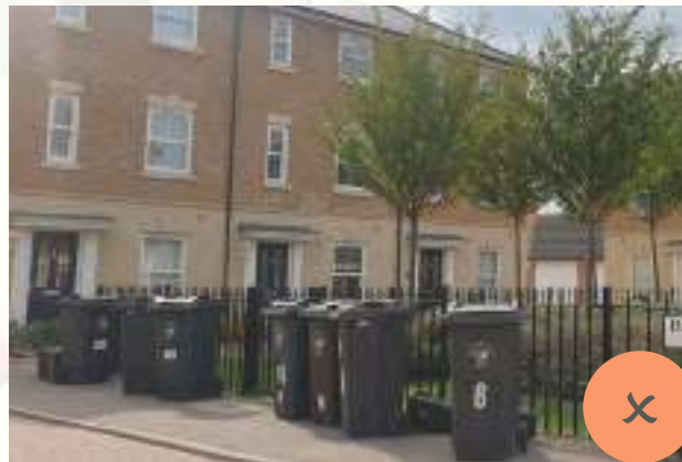
Poorly considered storage
