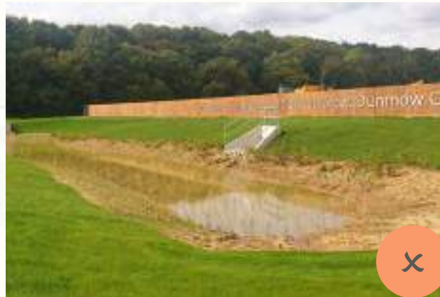
Water storage pushed to the edge of the site, providing little wider value
