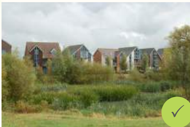
A new urban edge can be created on the northern boundary, overlooking the Carrant Brook River Corridor
