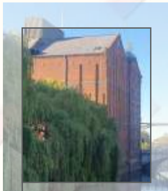
Large scale industrial buildings, close to
