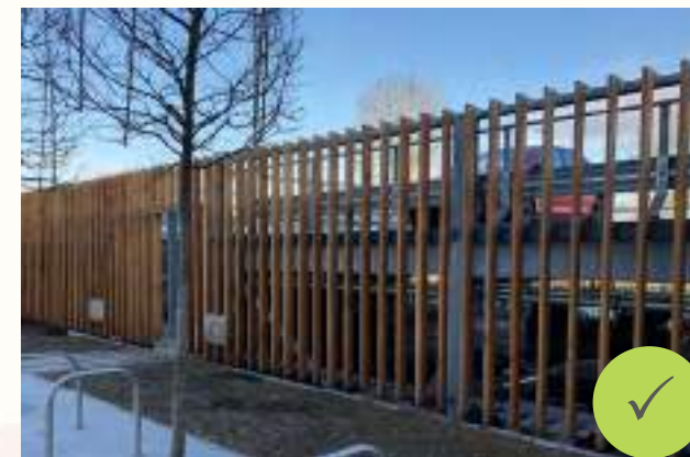
Car barns discreetly set into the landscape to limit their visual impact
