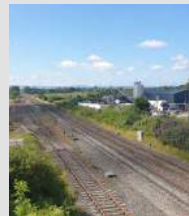
▲ The railway line, looking south from Ashchurch station
