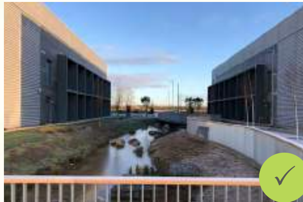
Using SuDS to support placemaking
