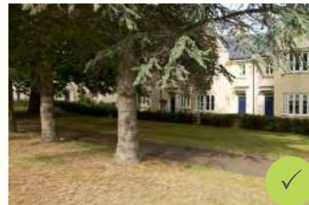
Homes overlooking an active travel corridor and the MoD site to the south
