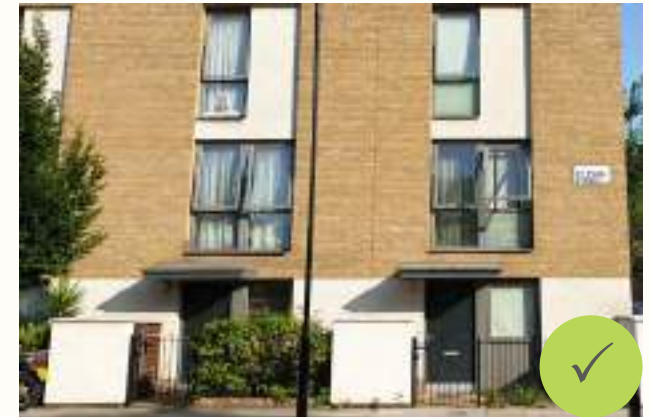
Carefully considered storage for bins, bikes and service meters
