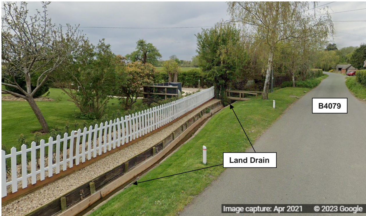
Photo 1: View of Land Drainage Ditch Parallel to B4079 Facing North-West
