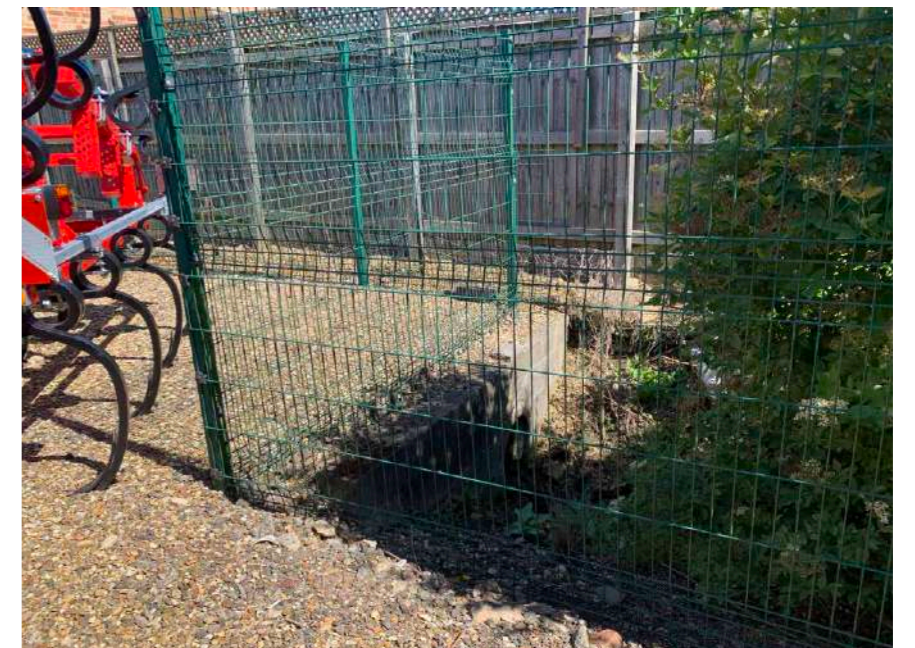
Existing drainage culvert in southern part of the site
