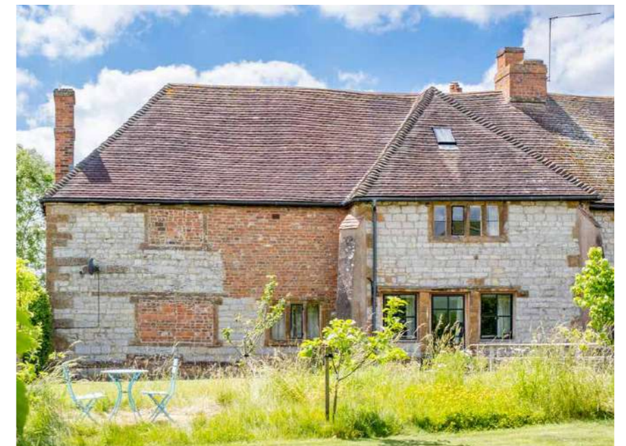
Gaydon Manor Farmhouse constructed of Stone, Brick & Tile
