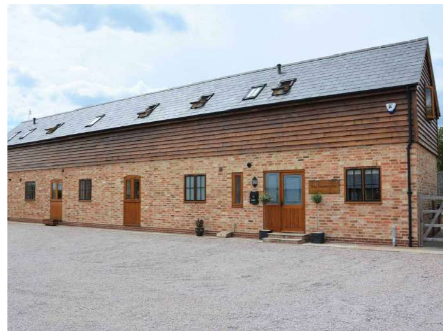
Brick, Timber & Slate Dwelling at Gaydon Farm Barns
