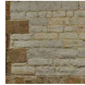
Coursed Lias Limestone with Ironstone detailing to match traditional local stonework
