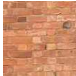
Pink/Orange Brick to match traditional local brickwork
