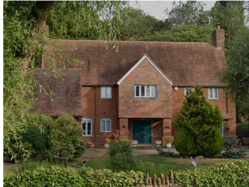
Brick dwelling with tile hanging along Kineton Road
