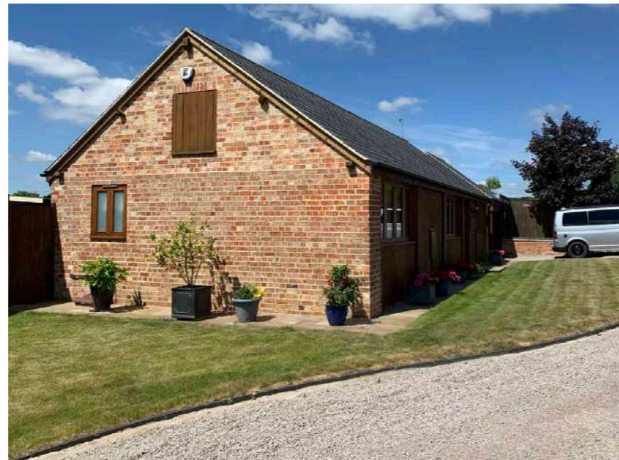
The Croft Bungalow Conversion
