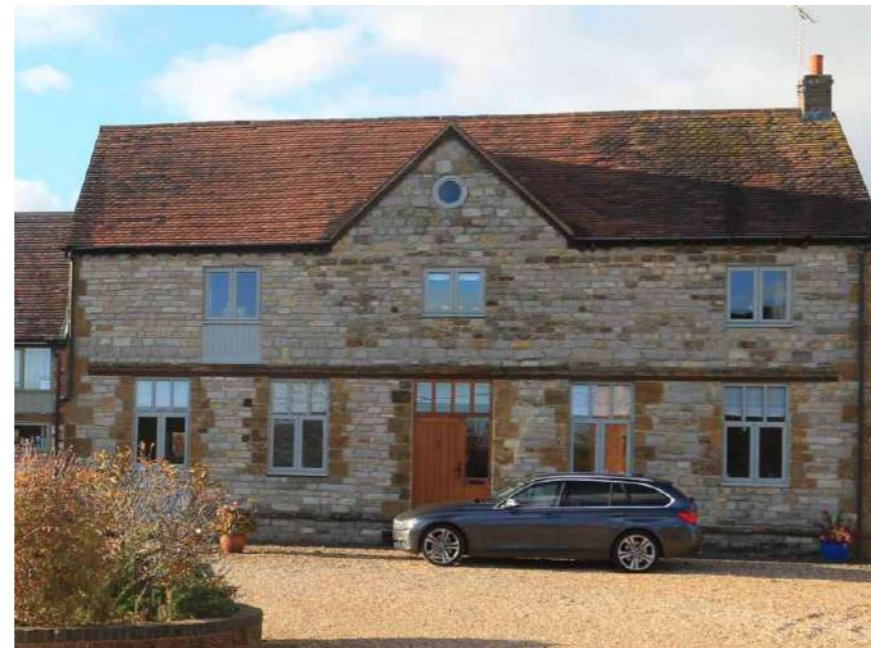
Stable at Gaydon Manor Farmhouse
