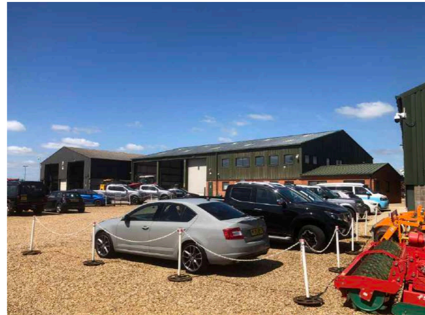
Central and western agricultural buildings
