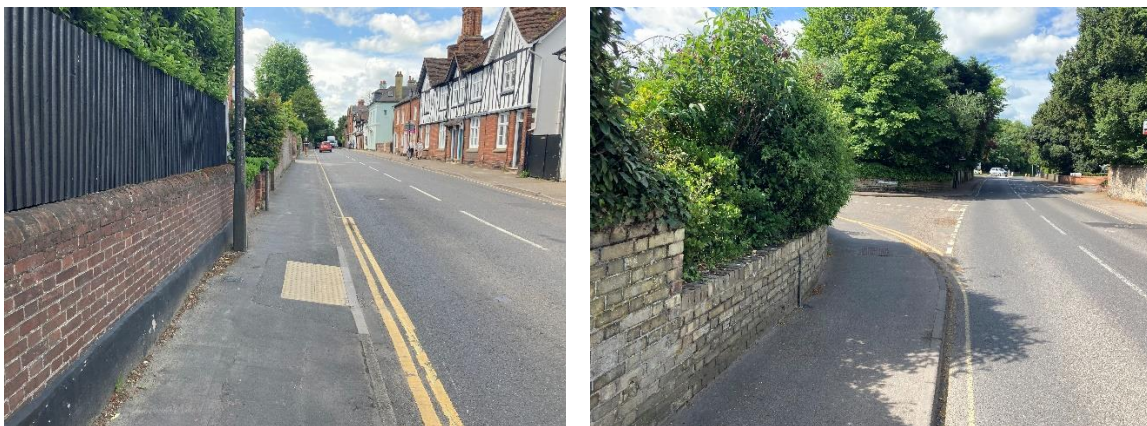
Figure 5.3: Footway on London Road and at Junction with Little Larchmount
