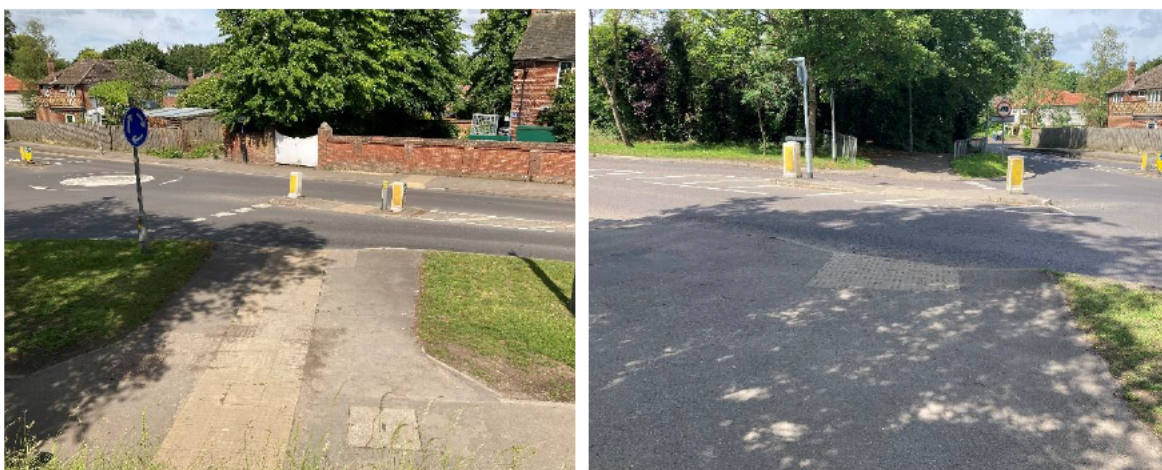
Figure 5.5: Uncontrolled Crossing Points at London Road / Newport Road Junction
