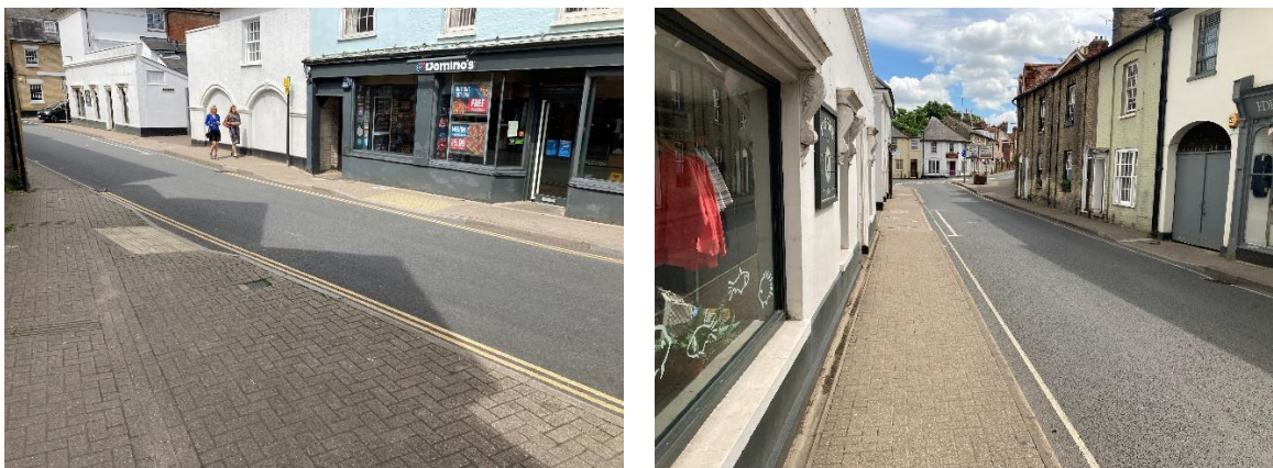
Figure 3.19: Footways on Hill Street
