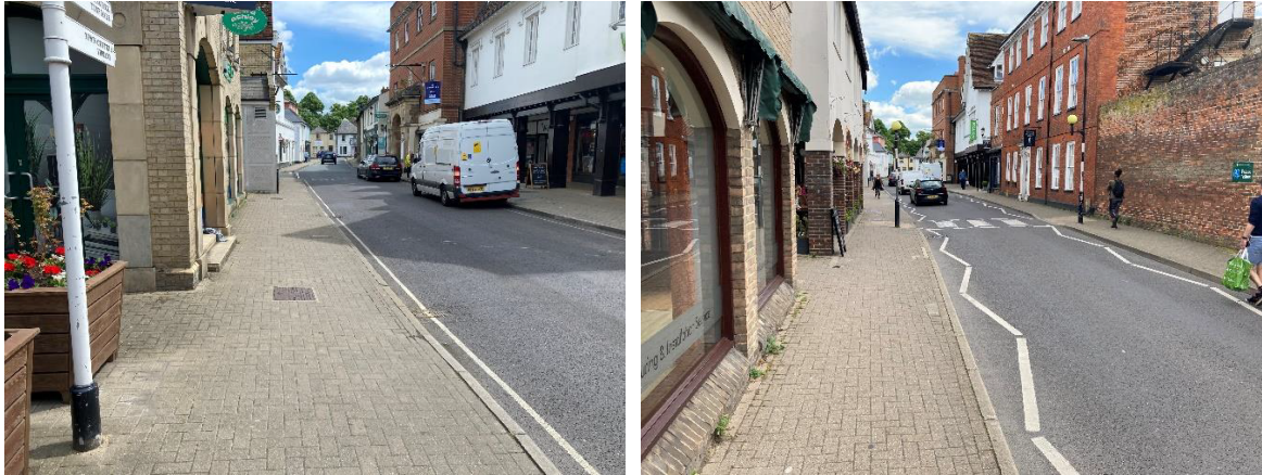
Figure 3.20: Footways on Hill Street to the west of Market Street including Zebra Crossing
