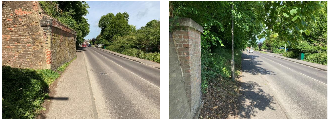
Figure 3.4: Restricted Footway Width and Overhanging Vegetation
