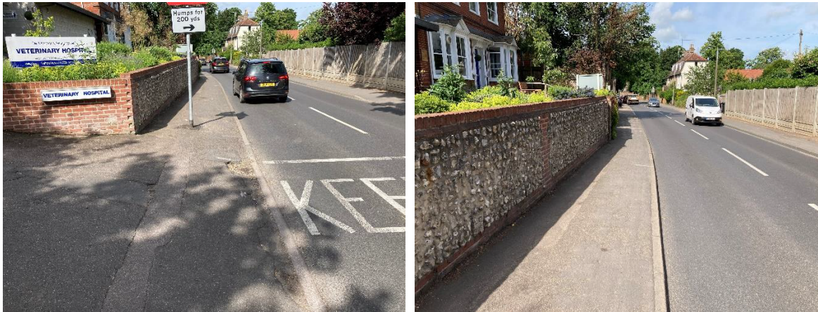
Figure 3.7: Sign within Footway and Pinch Point
