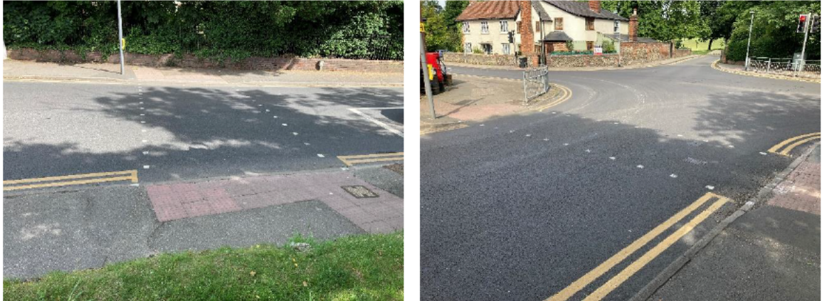
Figure 3.9: Crossing Facilities at Radwinter Road / Thaxted Road / Chaters Hill Junction
