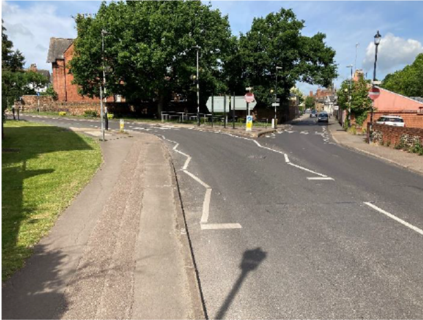
Figure 3.11: Zebra Crossings at Junction of East Street and Audley Road.
