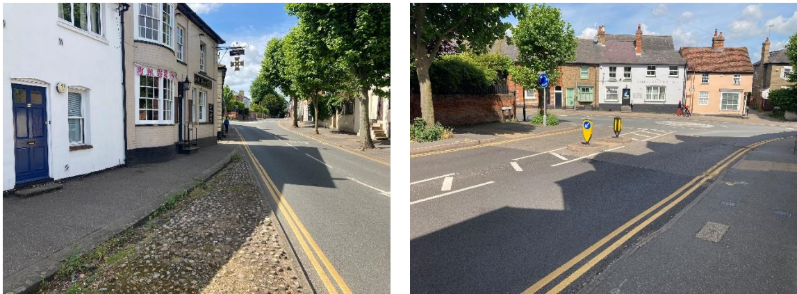
Figure 5.2: Footway on Debden Road and Crossing Point at Junction with London Road
