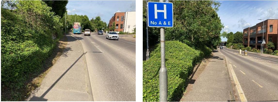
Figure 3.3: Encroachment of Vegetation and Lack of Tactile Paving at Crossing Point
