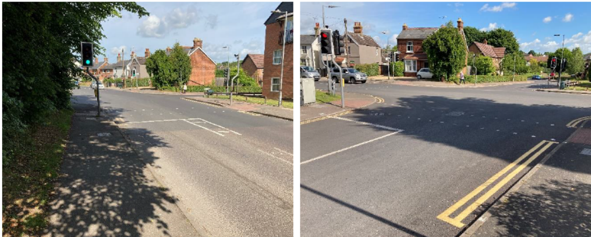
Figure 3.5: Controlled Pedestrian Crossing Facilities at the Junction of Radwinter Road / Elizabeth Way / Horn Brook
