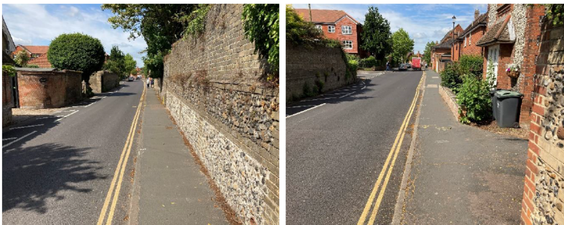
Figure 3.14: Limited Footway Width of Audley Road
