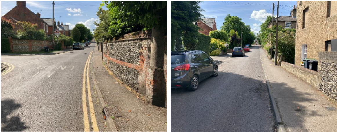
Figure 4.2: Footway on South Road
