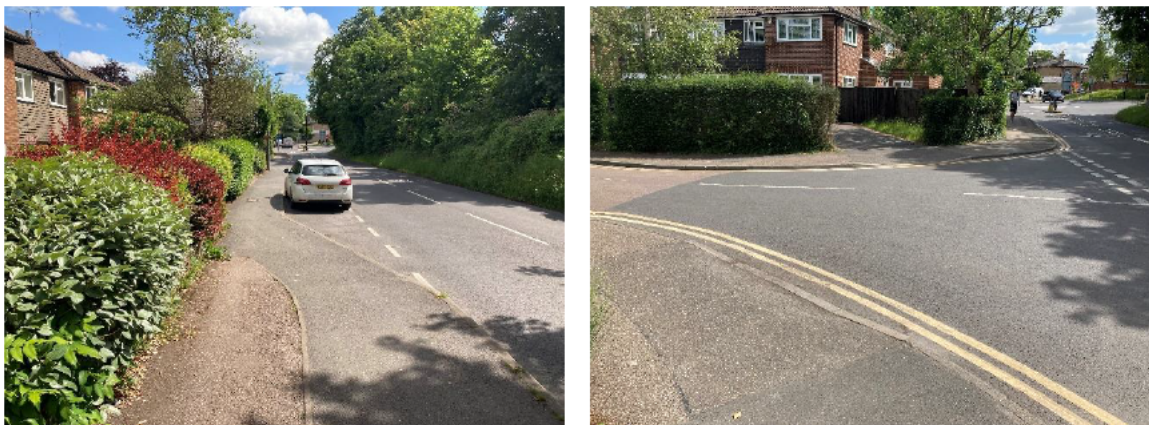
Figure 5.6: Footway on Northern Side of Audley End Road
