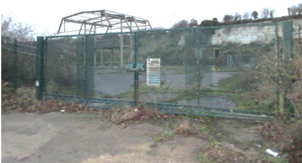
Plate 6: Fuel depot infrastructure, north of site
