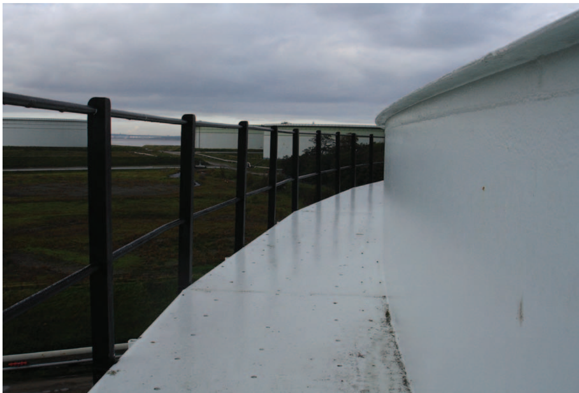
Figure 15 Top girder (walkway) on floating roof tank
