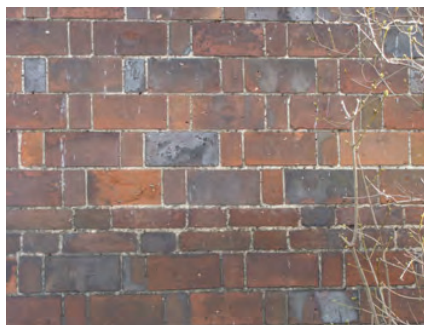
Picture 1.22 Prominent boundary wall in grounds of Elm Grove; unusual rat trap bonding
