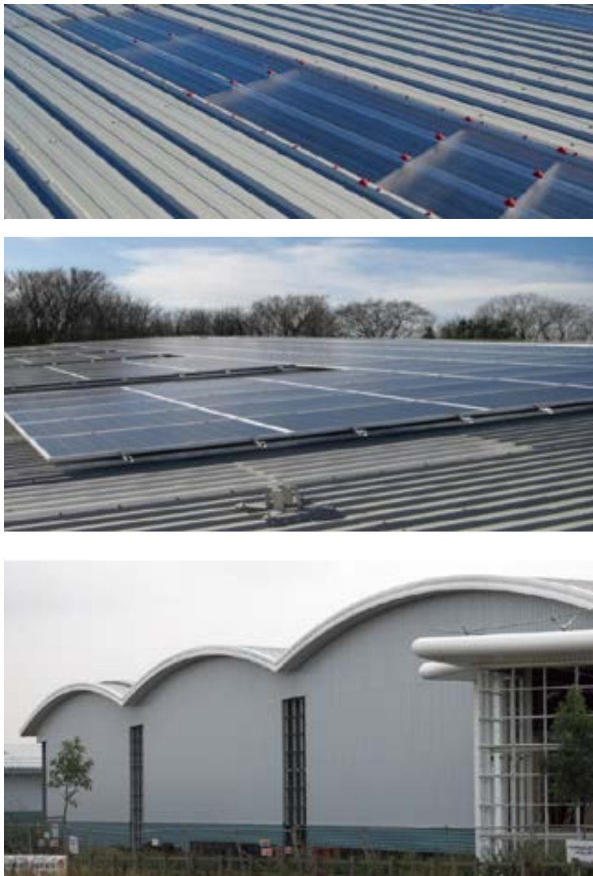
Low pitch curved roof with integrated in-plane polycarbonate rooflights and solar panels
