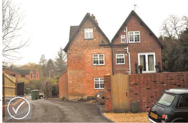
Driveway appropriate to the semi-rural context
