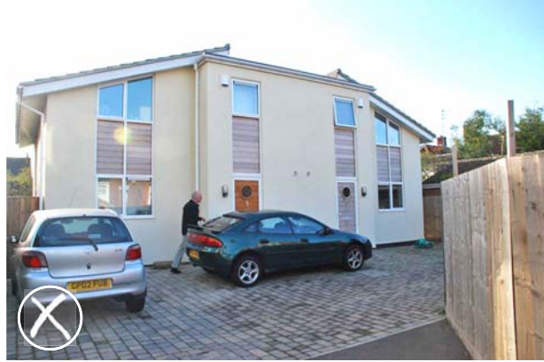
Rear garden development on a small plot - close in proximity to rear of existing dwelling, feels cramped and risks overlooking.
