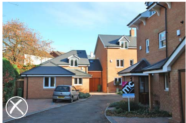
This space is perhaps too enclosed and the building on the right feels too high for the small space.
