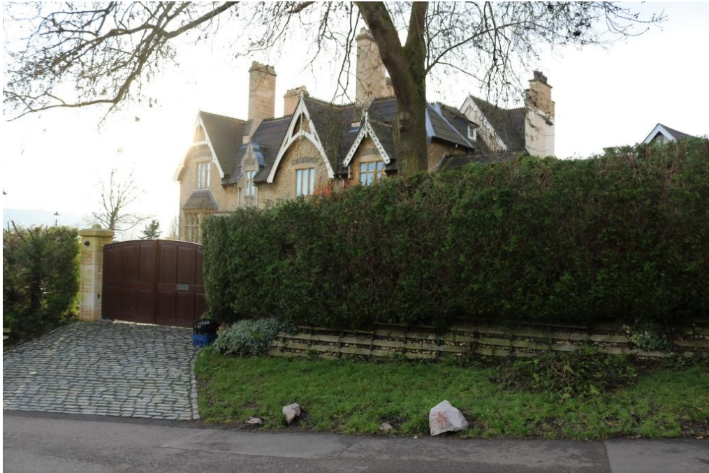
Plate 21: View of the Ashley Road frontage (east elevation) of Charlton Manor, showing its steeply pitched gables, decorative barge boards, tall chimneys, mullioned windows and 'crazy' pattern limestone wall facing. Note high conifer hedge screening the property from public view.
