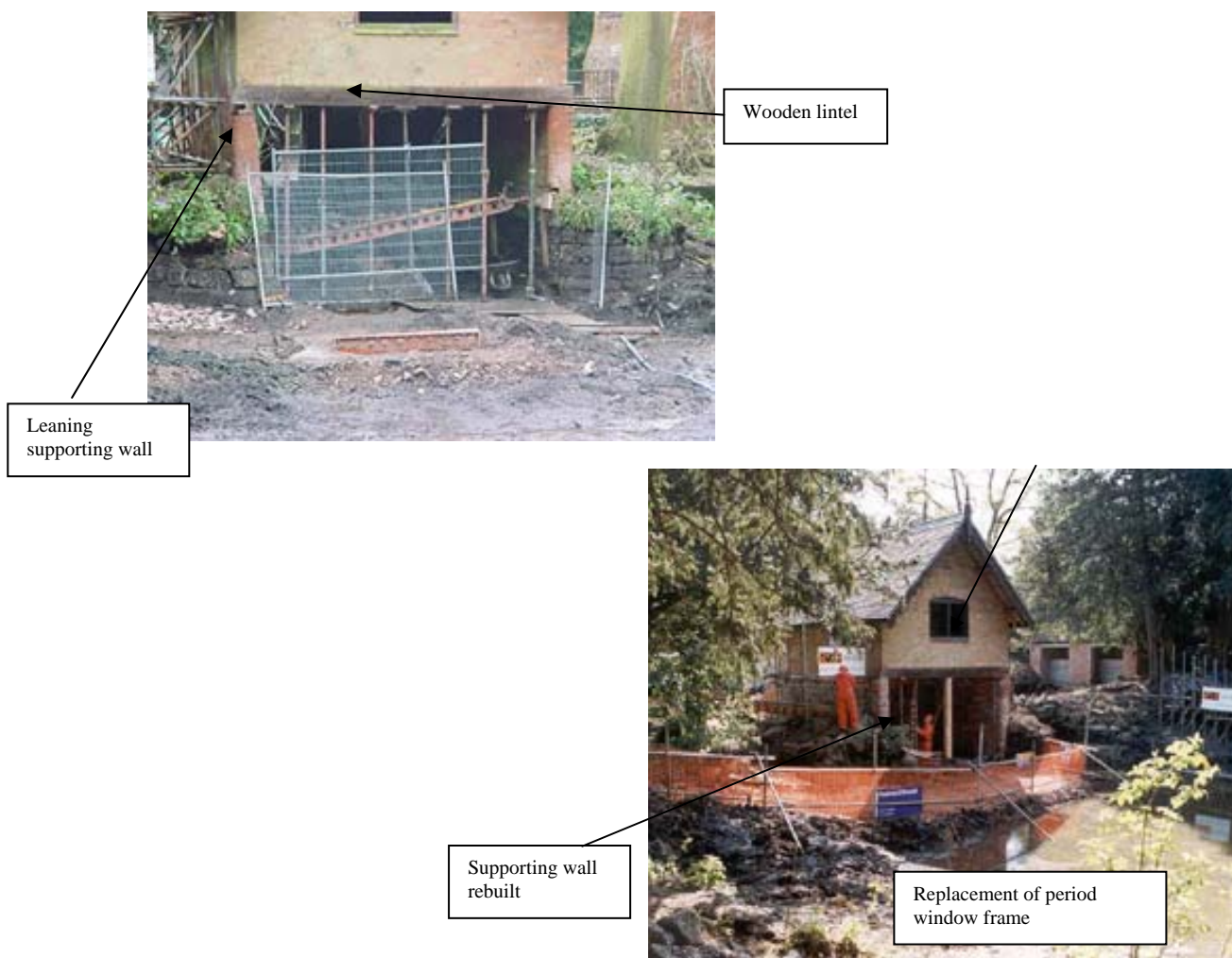
Figure 9.2.2 Restoration in progress
