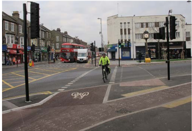
Figure 10.26: Circulating Cycle Stage Junction, Waltham Forest
