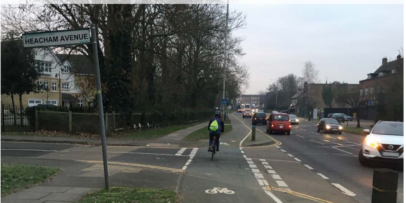
Figure 10.16: Partial set back, marked priority crossing, Hillingdon
