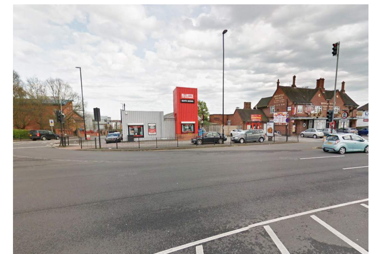
B. View from the Roundabout
