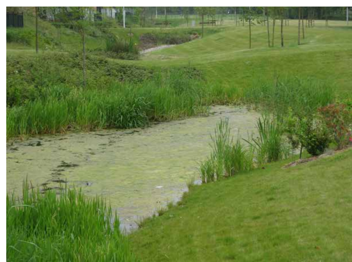
Sustainable drainage feature
