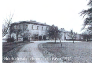
North elevation from north-east c.1971
