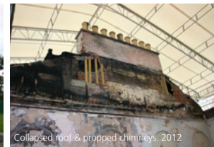
Collapsed roof & propped chimneys. 2012
