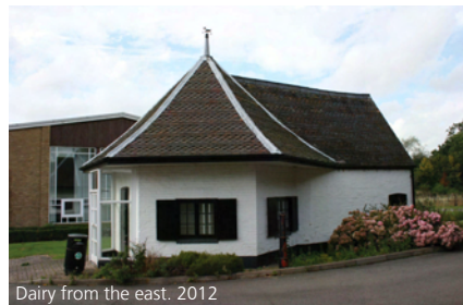
Dairy from the east. 2012
