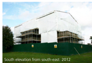
South elevation from south-east. 2012
